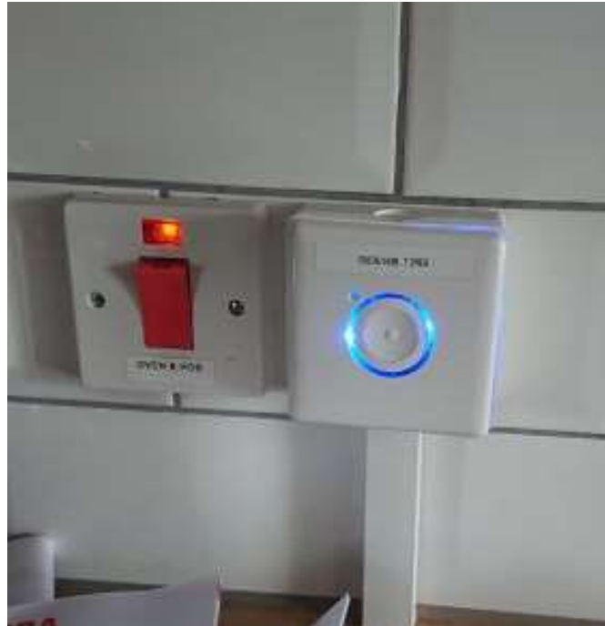
Example of a timer switch to minimise fires in cookers and hobs
